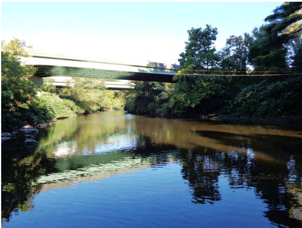
Figure 3 Station NN12 upstream – I-190 Bridges (9/24/2013)
