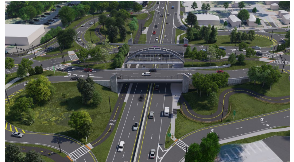
Route 27 over Route 9 Modified Diverging Diamond Interchange
