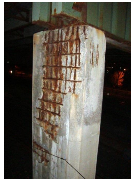
Deteriorated concrete column supporting the I-90 viaduct
