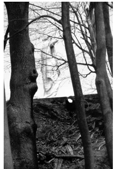
Corrugated metal pipe at the concrete curb on the circular drive
