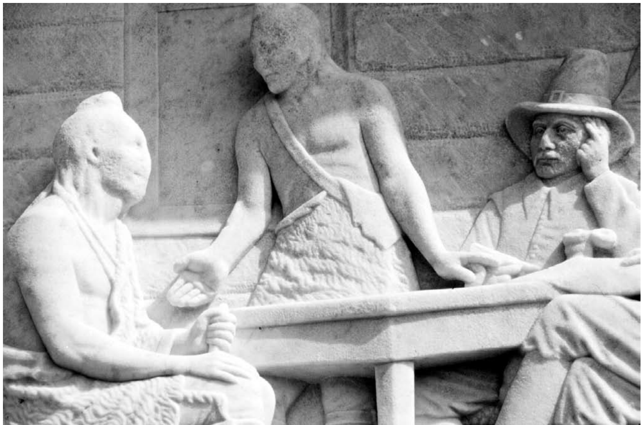
Detail of erosion at bas-relief
