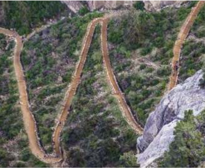
Switchback Trails A trail that cuts sharply back and forth to traverse steep topography, breaking the path into multiple lesser-degree slopes.
