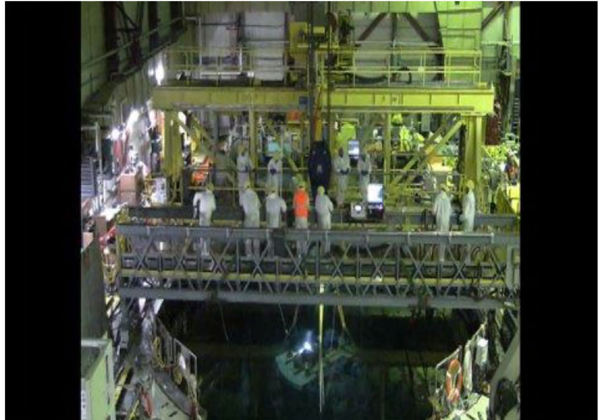
Installation of shroud segmentation tooling
