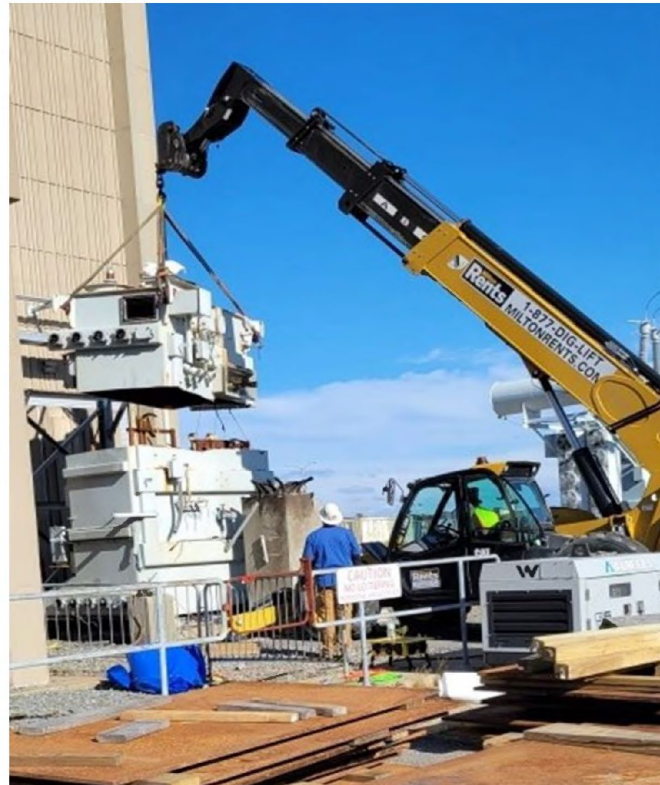
Main Transformer Removal
