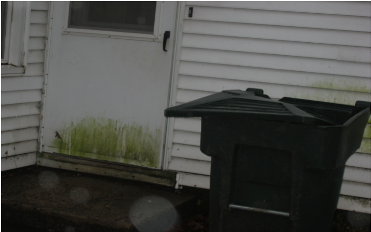
200-1 Development, Linden Street – Mold on Entrance Door and Siding
