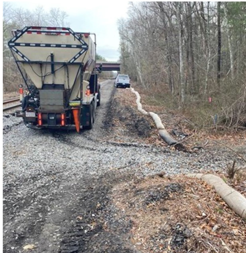
Erosion controls along the ROW
