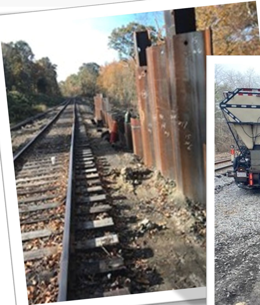
Ongoing sheet pile detail work
