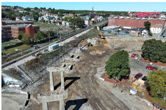
Image 3. Ramp C Demolition
