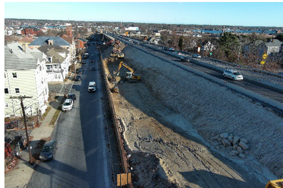
Image 4. Excavation along Ramp A
