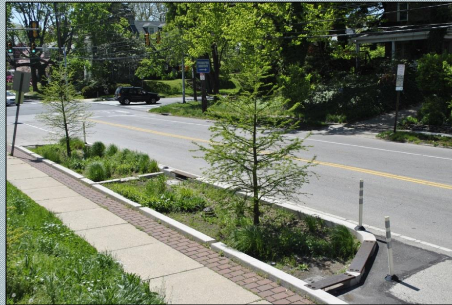
Contained bioswale or planter box
