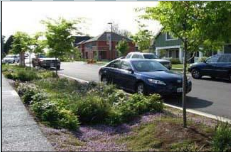
Bioswale between sidewalk and street
