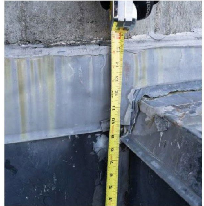
Photo 221 – Deteriorated flashing and parapet connections at west stair tower are typical.
