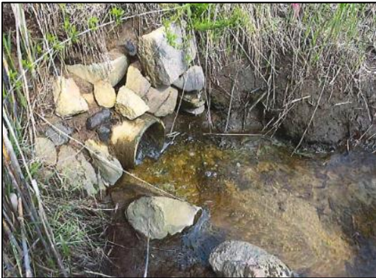
Before: Undersized 12" tidal culvert under Crosby Lane
