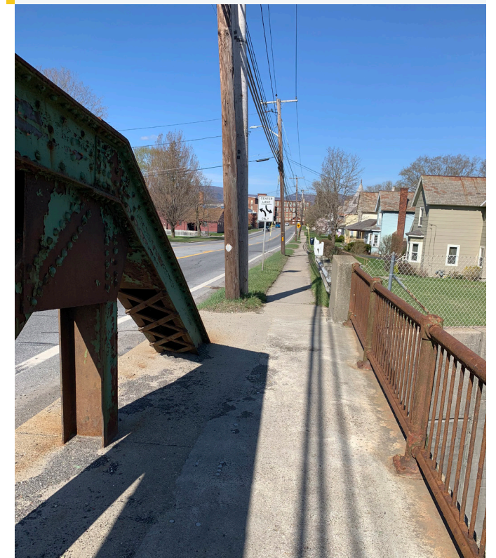
Figure 39 —Existing trusses and sidewalk on Hoosic River bridge
