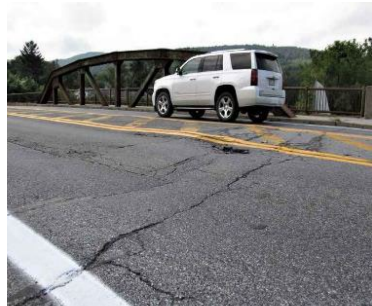
Bituminous concrete wearing surface showing signs of cracking and spalling
