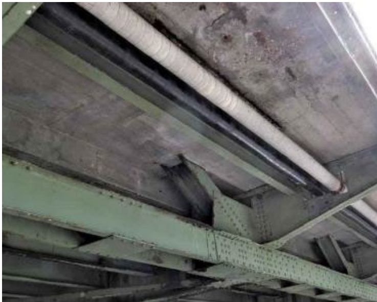
Utility Conduits beneath the bridge
