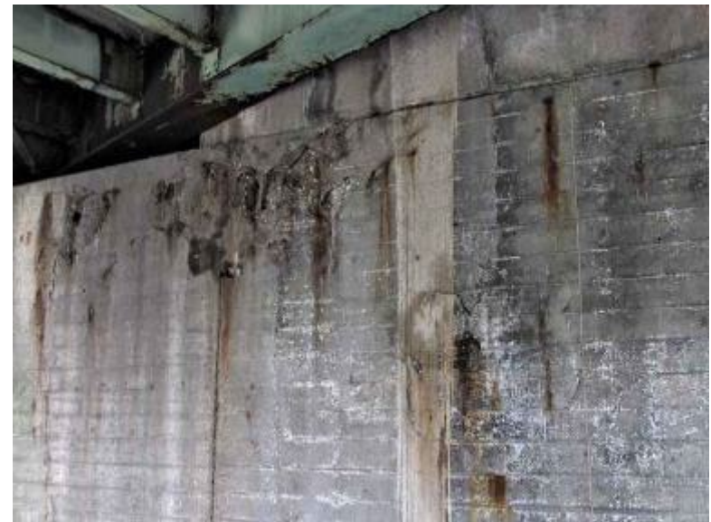
Spalling at West Abutment
