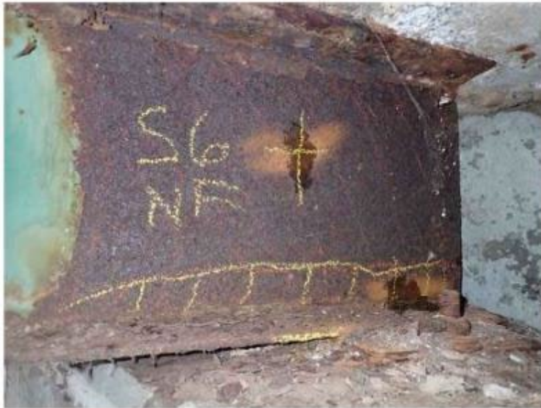
Section loss in truss stringer
