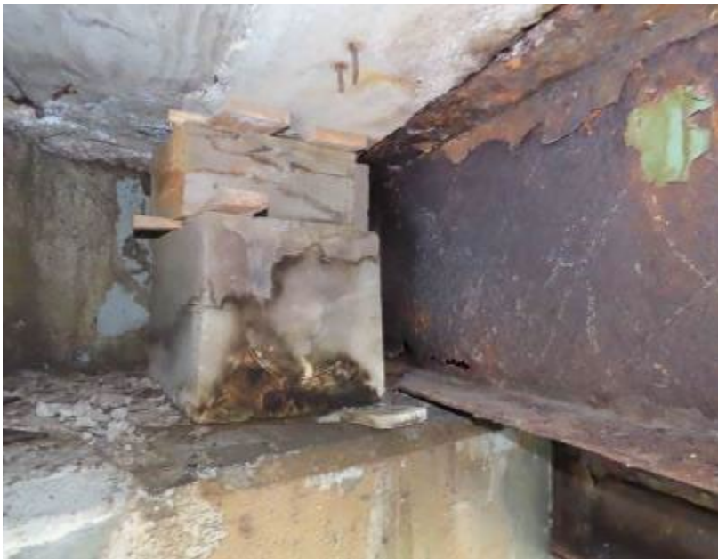
Stringer section loss and installed cribbing
