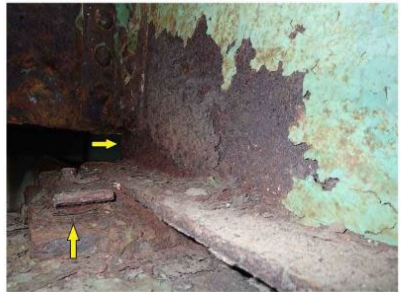
Web buckling and pack rust around the bearings
