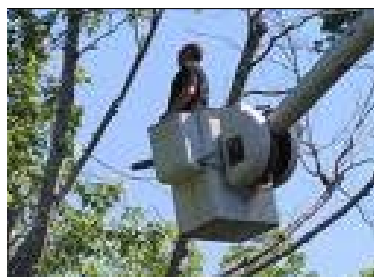
Tree-pruning to Protect Utility Lines
