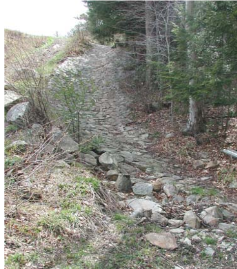
Lower section of spillway (dry)
