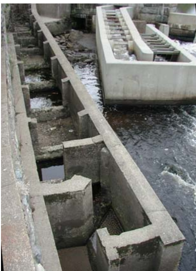
Old (left) and new (right) fishways at Ipswich Mills Dam
