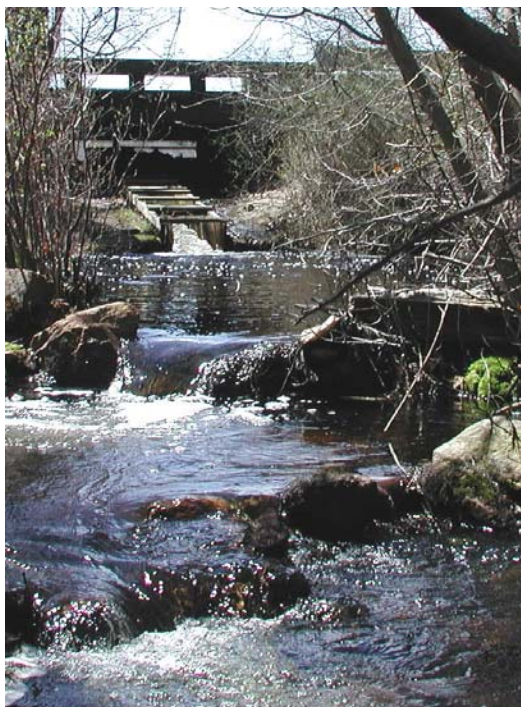
Stream baffles and denil ladder at Lily Pond
