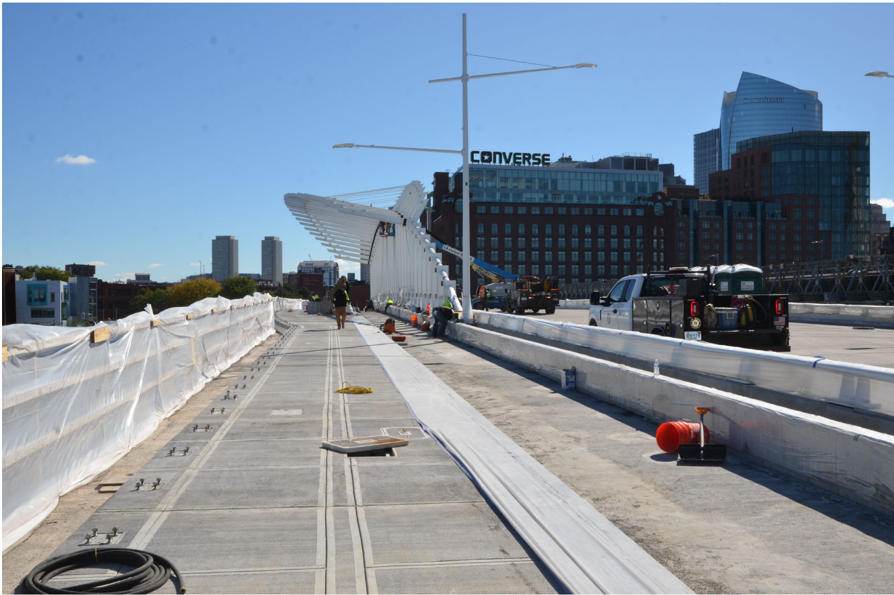
East sidewalks, barriers, and bridge rail complete
