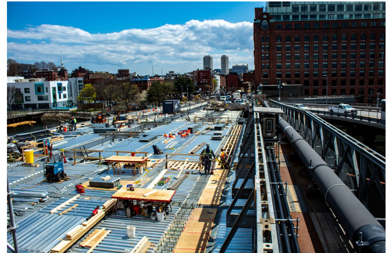
Deck formwork installation
