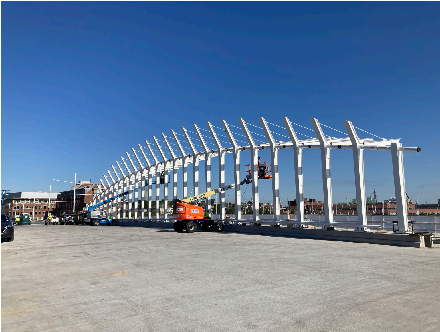
East architectural trellis installation
