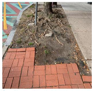
Tree well in poor condition with missing bricks
