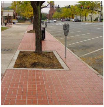
Example of Perma-Cast Shake-On Color Hardener, Basketweave Stencil (Source: https://www.butterfieldcolor.com/gallery/stenciled-concrete/)
