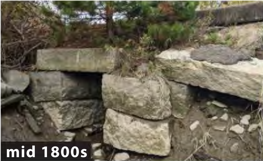
Quarried and shaped granite blocks at culvert opening underneath and associated with Saugus Branch Railroad.
