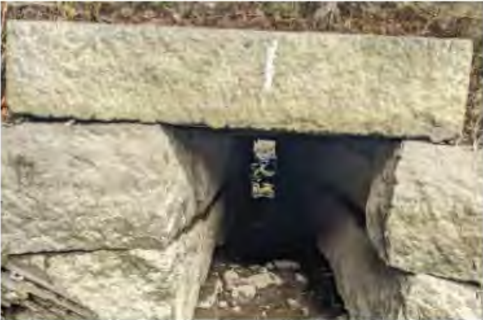
Closeup of culvert (in excellent condition); quarried granite had 3/4" drill marks consistent with post 1830s stone quarries.
