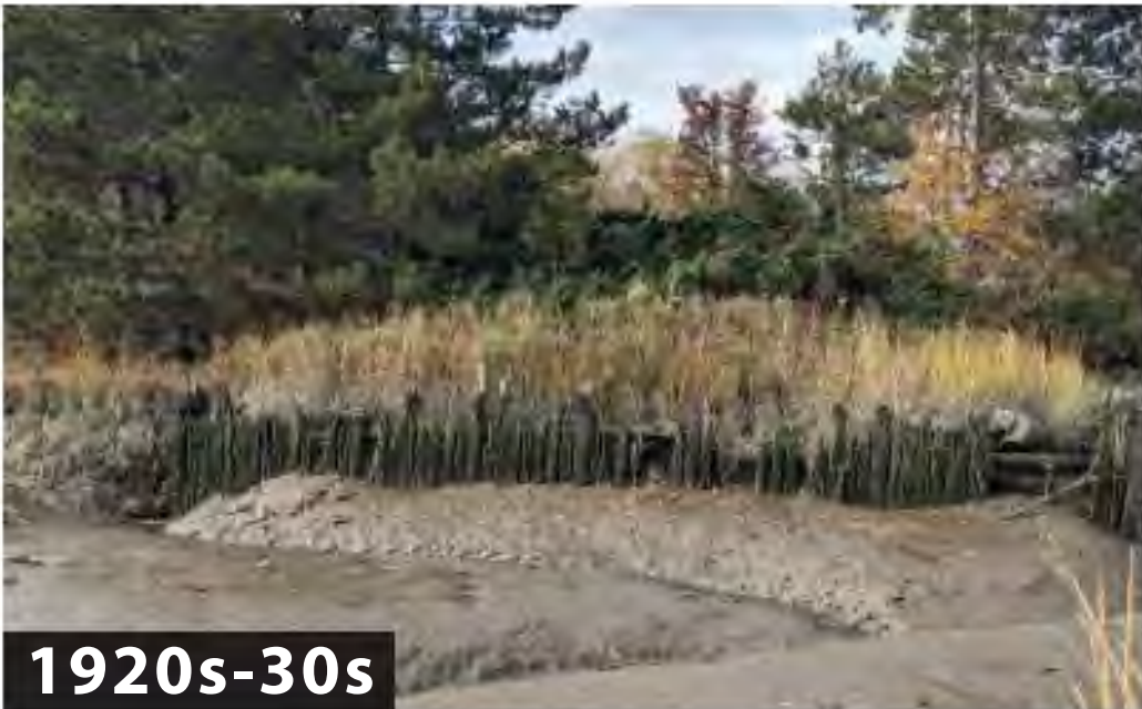
Plank retaining wall/fencing for erosion control at low tide, assumed association with the Universal Tide Power Co.
