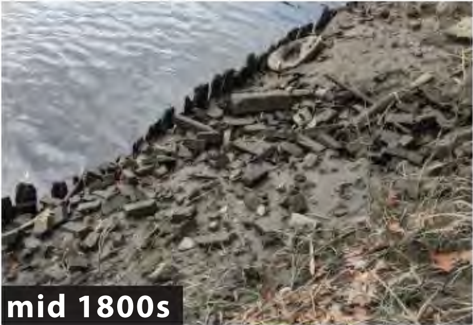
Brick and other backfill at plank retaining walls, potential remnants from Newhall Brickyard.
