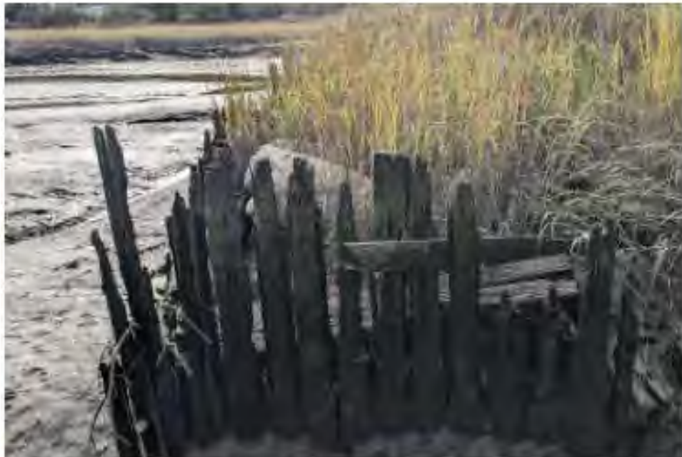
Closeup of wood plank fencing for erosion control.
