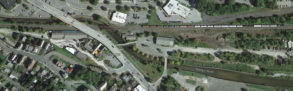
Figure 3.6: North Adams, MA yard – Google Earth
