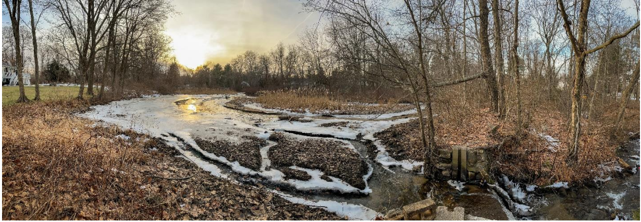
Mill Pond prior to dam removal. January 2022. PC: Sterling Worrell
