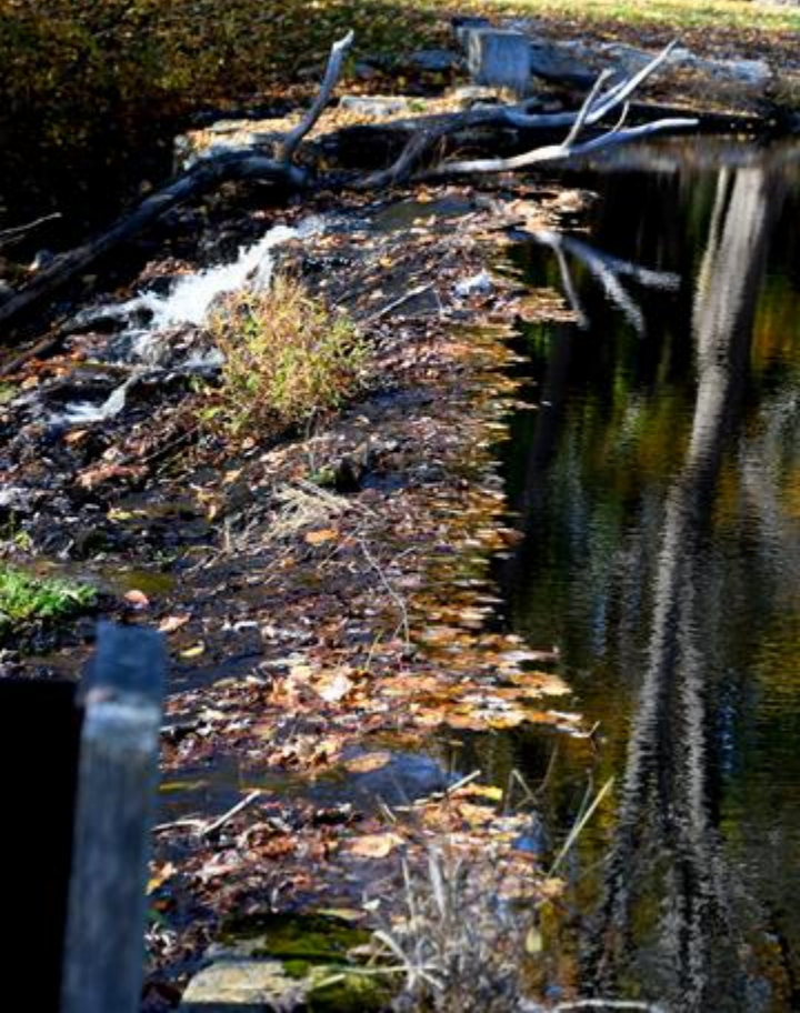
Tisdale/Assonet River Dam Elm Street, Assonet Dam November 1, 2024
