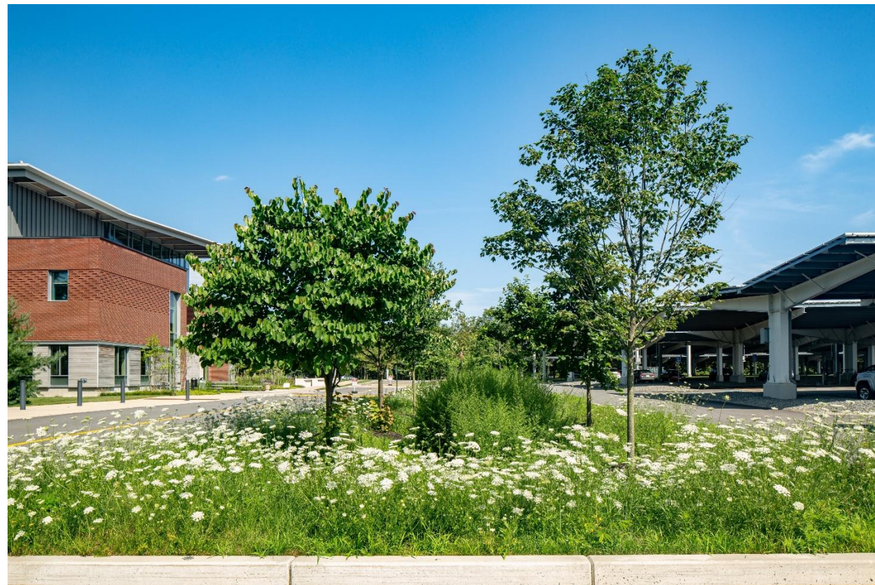
Bristol Community College : John J. Sprega Health and Science Building
