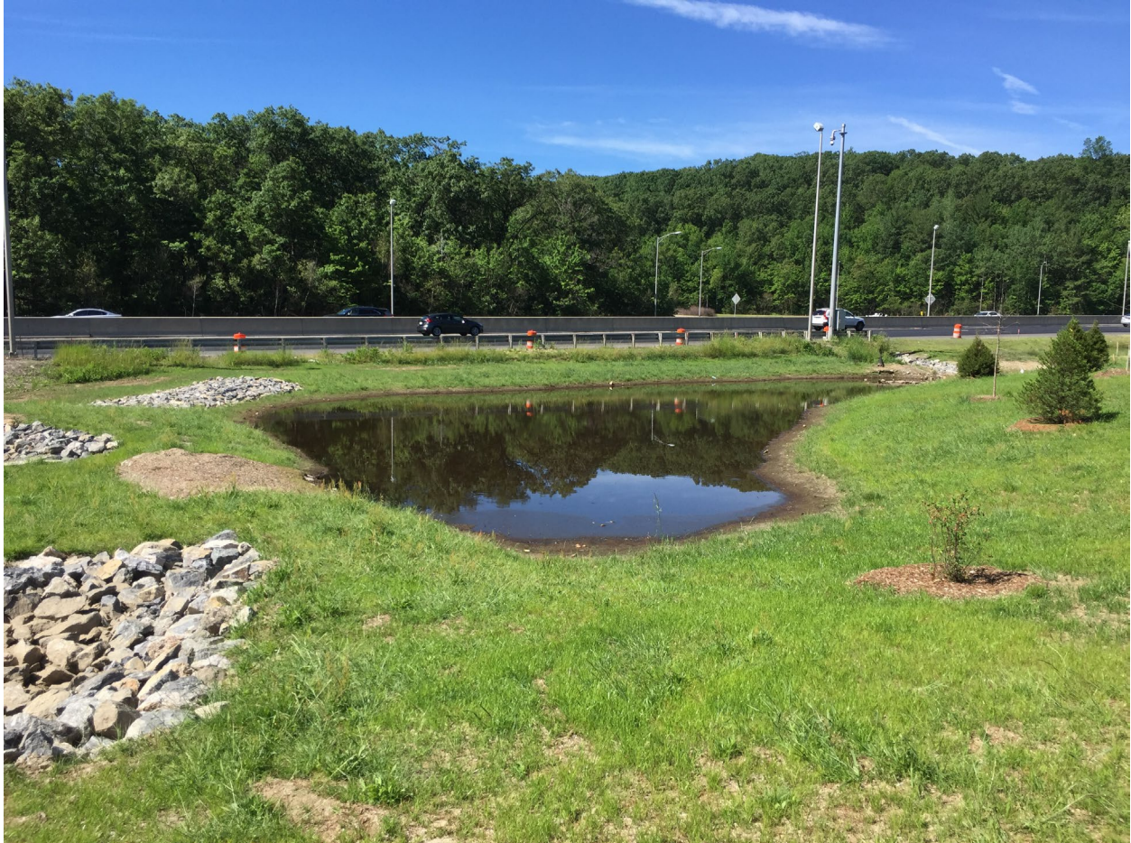
Infiltration Basin on I-90 treating stormwater discharge to Dorothy Pond in Millbury, MA.
