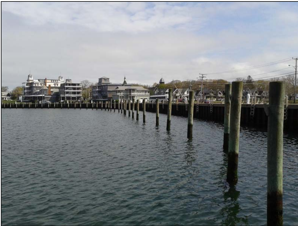
Figure V-2. View of Oak Bluffs Harbor main basin bordered by a vertical sheet-pile bulkhead.
