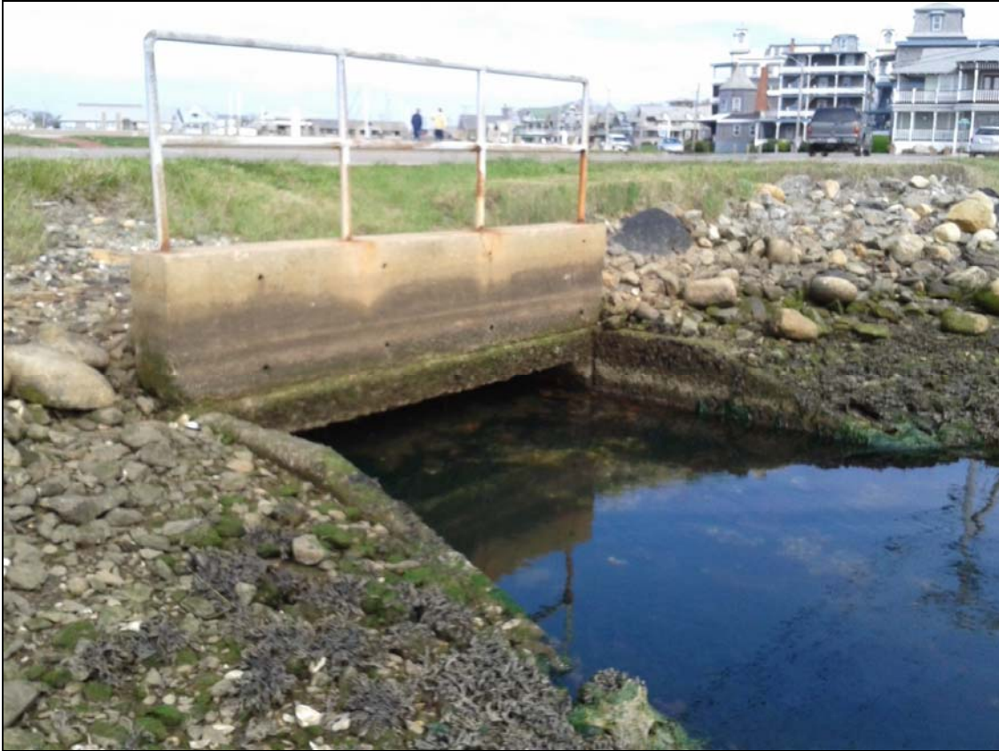
Figure V-10. View of Sunset Lake box culvert to Oak Bluffs Harbor, from the pond side.
