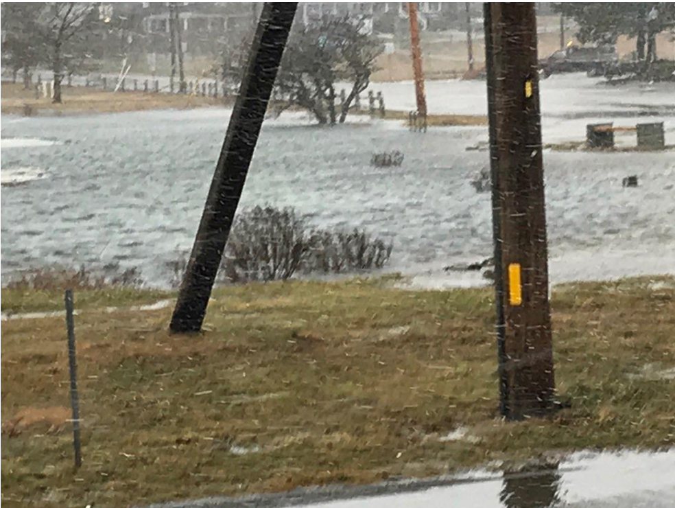
FIGURE 2 FLOODING AT LAKE AVENUE PUMP STATION
