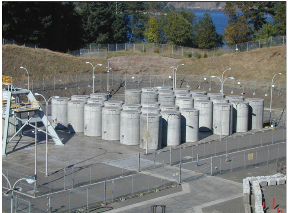
Figure 4: Spent Nuclear Fuel in Dry Storage
