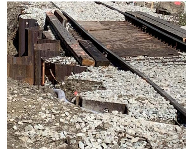
Cofferdam Installation
