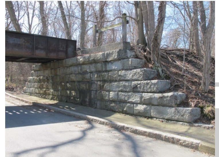
Collins Street, South Abutment and Drainage Trough
