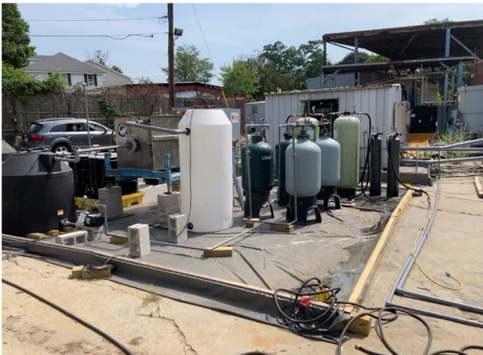
LGAC VOC treatment system components
