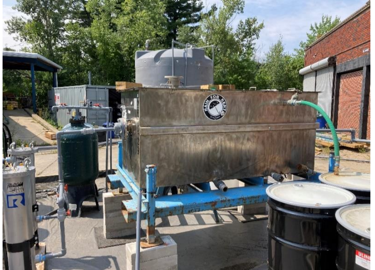
Oil/Water Separator & oil storage drums
