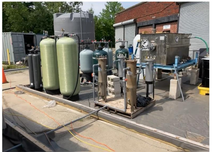
LGAC PFAS treatment system components
