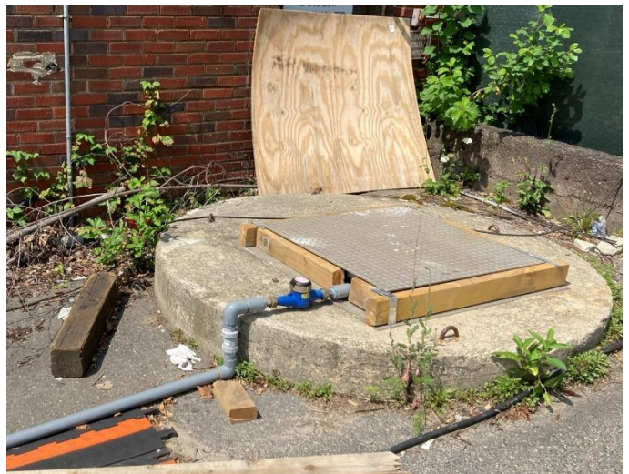
LGAC system discharge to sewer manhole
