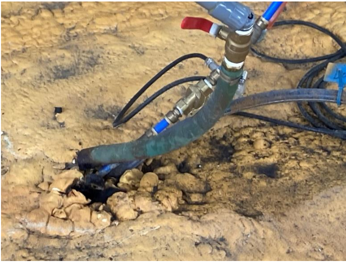
Close-up of vapor, drip & power lines @ electrodes
