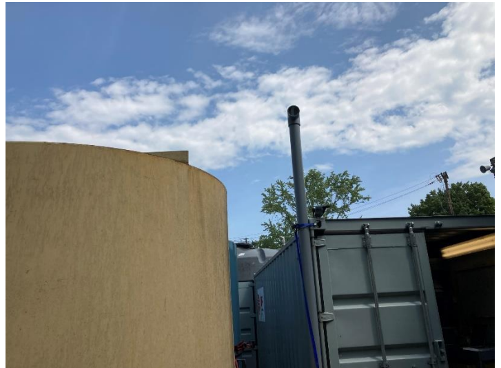
VGAC System Discharge Stack
