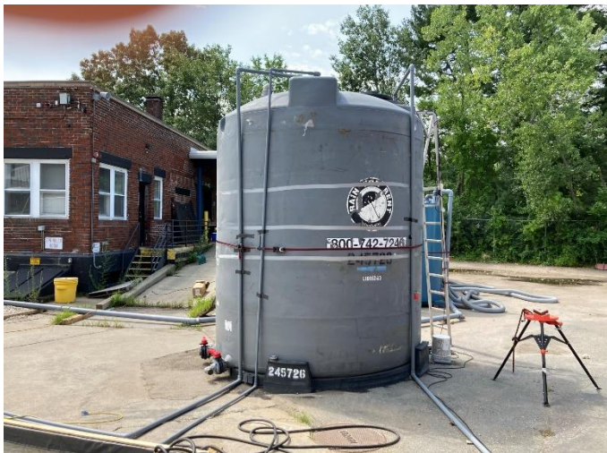
LGAC system 7000-gallon holding/discharge tank
