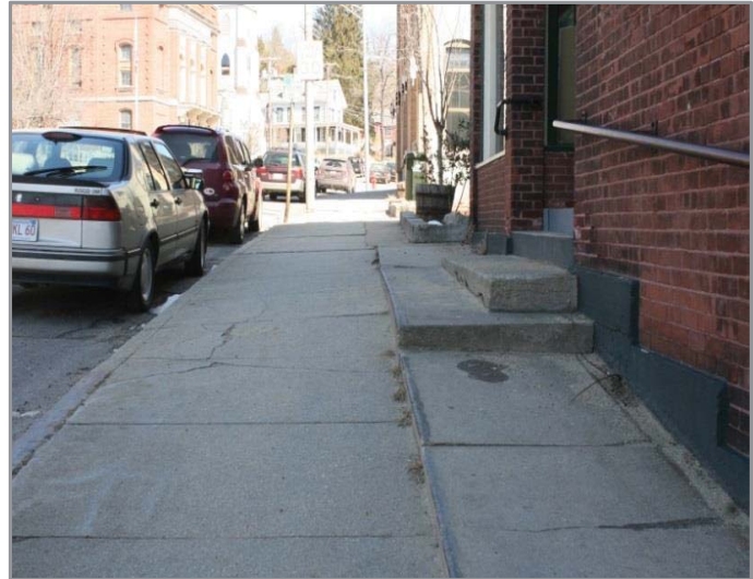
The sidewalk on the east side of North Main Street is uneven and there are tripping hazards.
