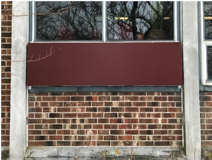
Photos 3 and 4 – Outdoor Air Intakes Boarded Over
