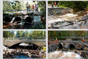
Clickwheel from top left: First replacement culvert (2010), culvert/bridge culvert failure due to flood (from time 2011) "emergency temporary replacement" culvert (2011), replacement bridge (2016).
