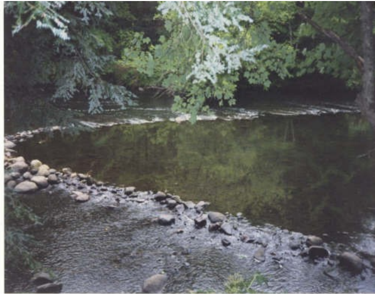
Arc of weir visible in low water conditions.
