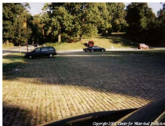
The use of alternative pavers in overflow areas reduces impervious surface coverage and helps facilitate groundwater recharge. Credit: Center for Watershed Protection
