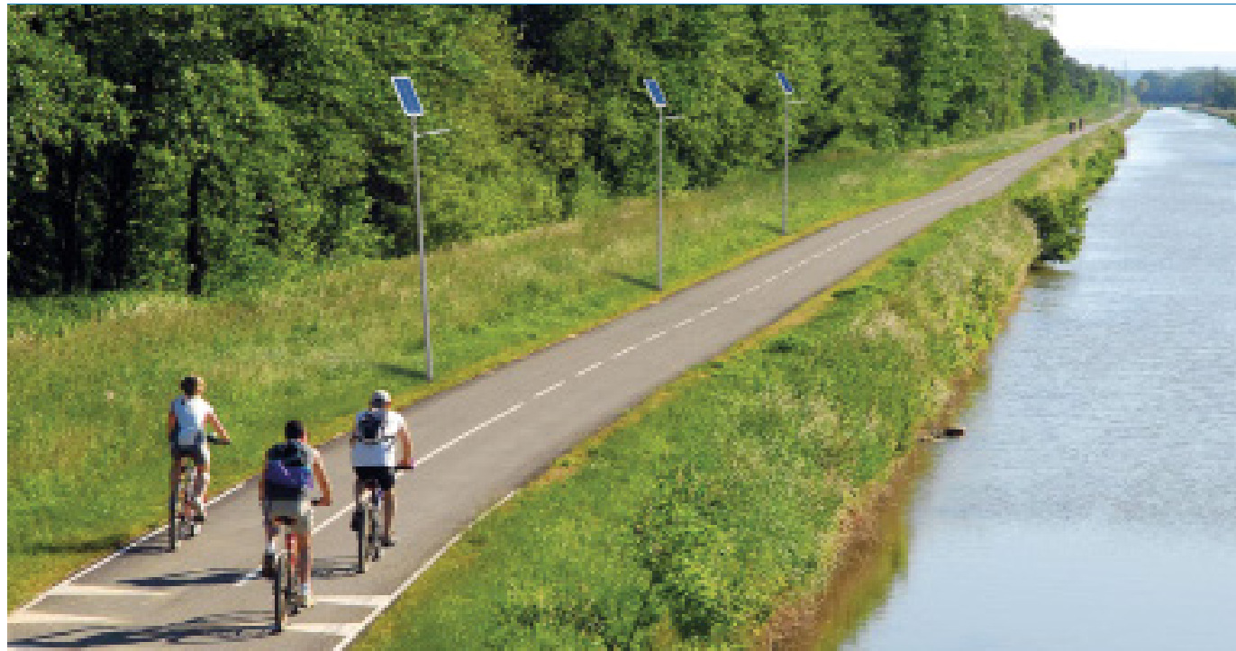
Figure 3-39. Example of a shared use path with solar lighting.
