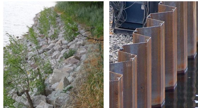
New Canal Wall & Riverstone Slope
