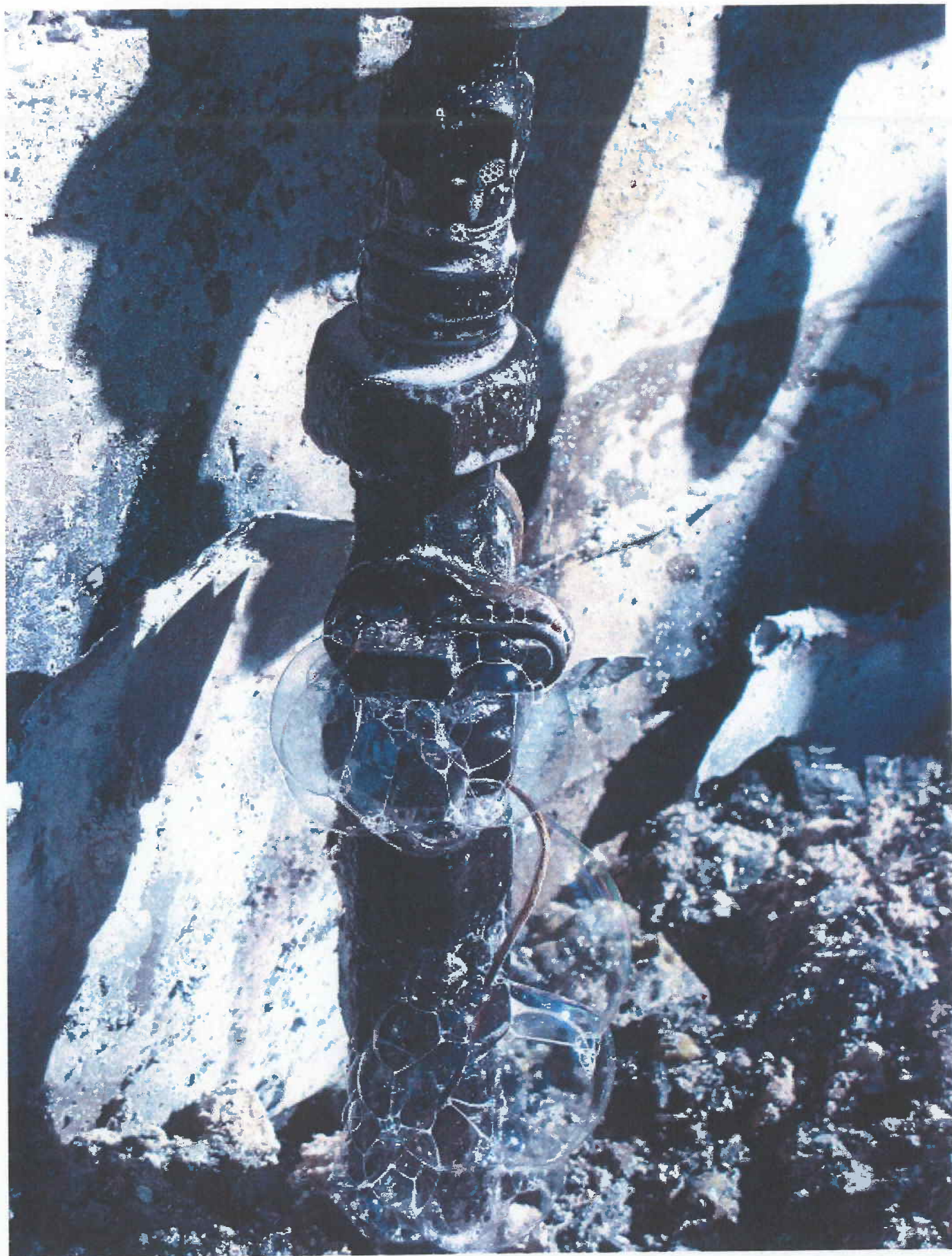
Service Riser Valve and Insulating Fitting
