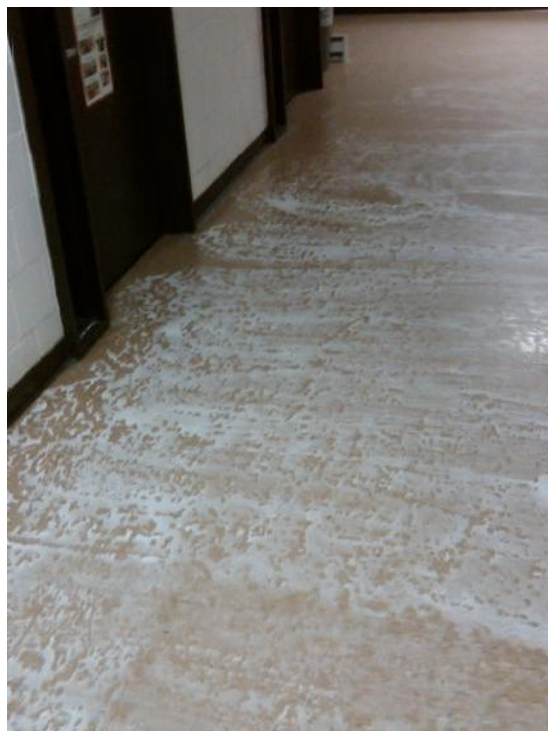
Corridor with applied "HgX ® " neutralizing agent
