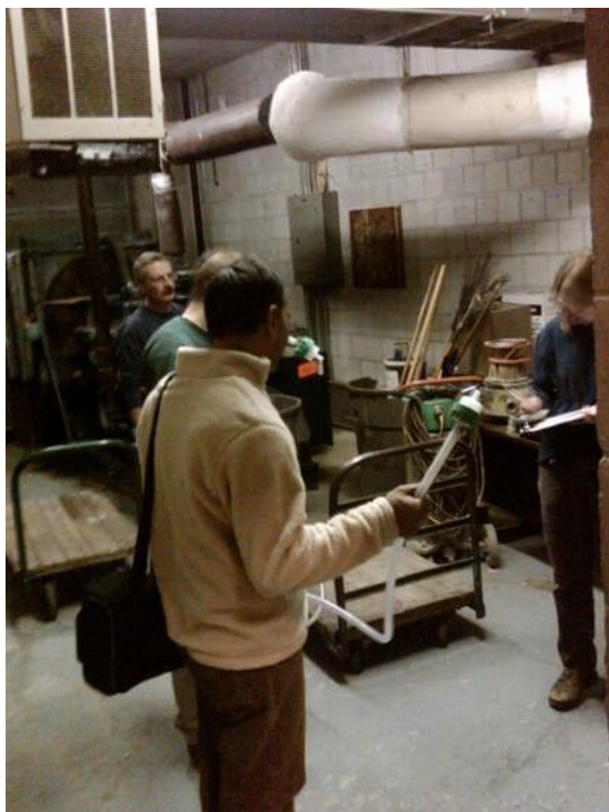
Mechanical Storage Room – Testing Air with Lumex Meters
