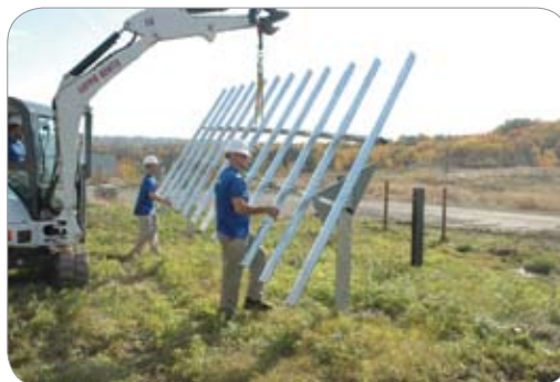
Figure 6: Driven Pile Mounting Structure (photo: Solar FlexRack)
