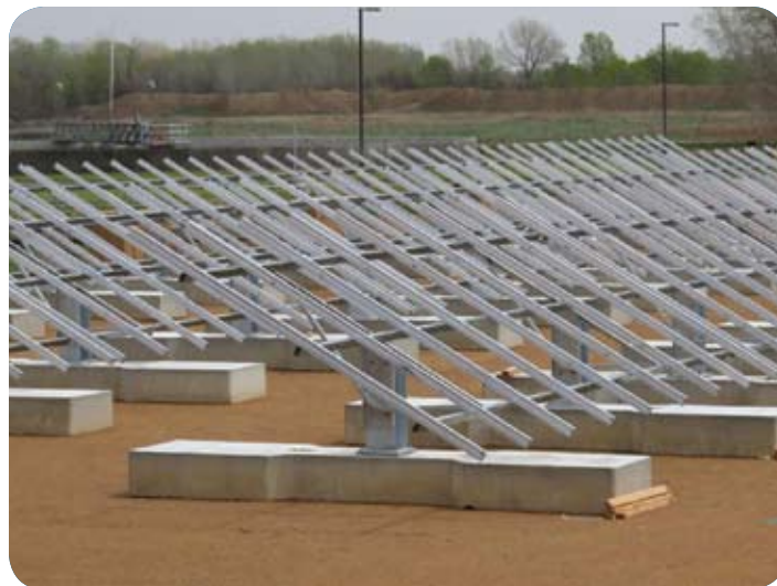
Figure 5: High-density Pre-cast Concrete System (photo: Solar FlexRack)
