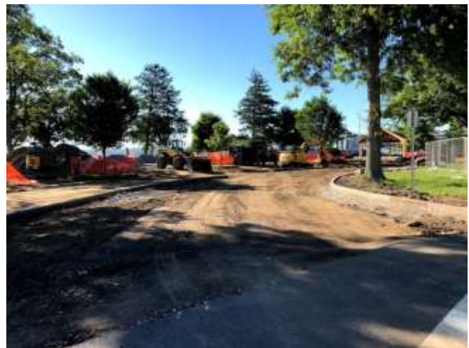
Pathway grading underway, drainage installed and curbs reset in parking pullout
