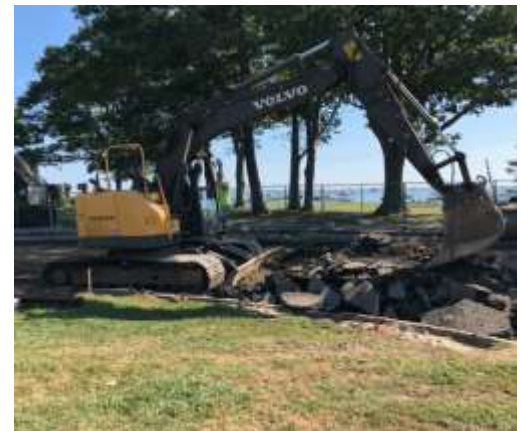
Below: Breaking ground at North Park parking area
