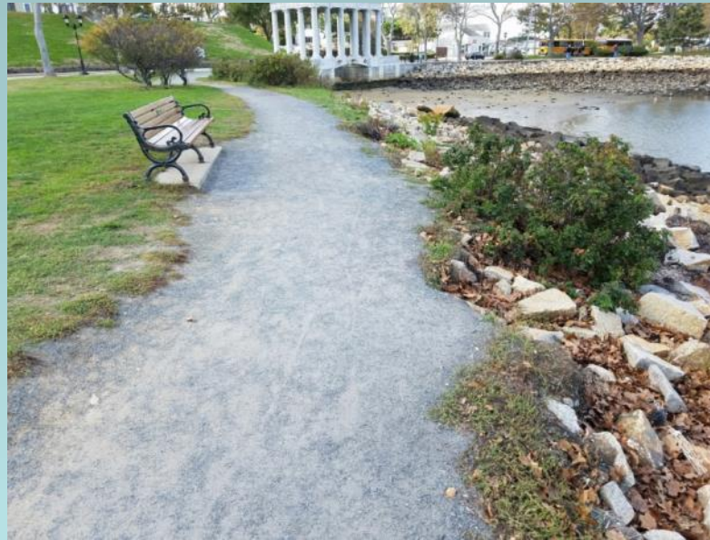
Localized collapse at rip rap
