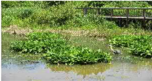
Floodwater Detention and Retention Basins
