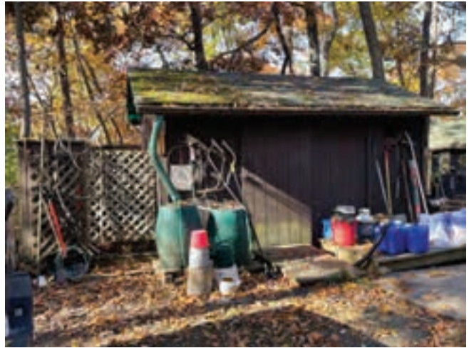
Figure 2-45. Sheldon Cabin's accessory storage shed showing cisterns for non-potable rainwater collection. Also shown are potable water jugs for drinking water and a propane tank used for heating/cooking.
