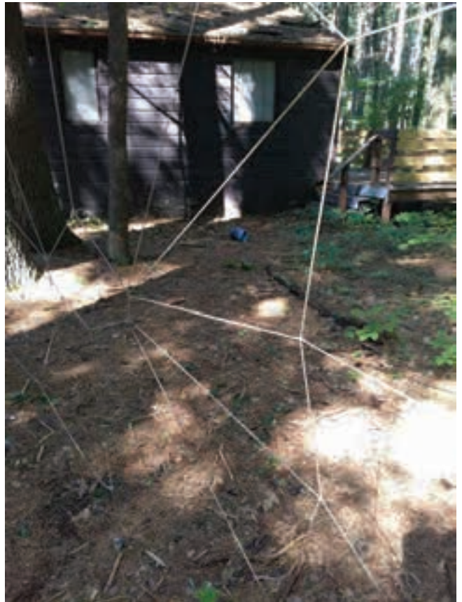
Figure 2-80. Surfacing and ropes course are not safety compliant
