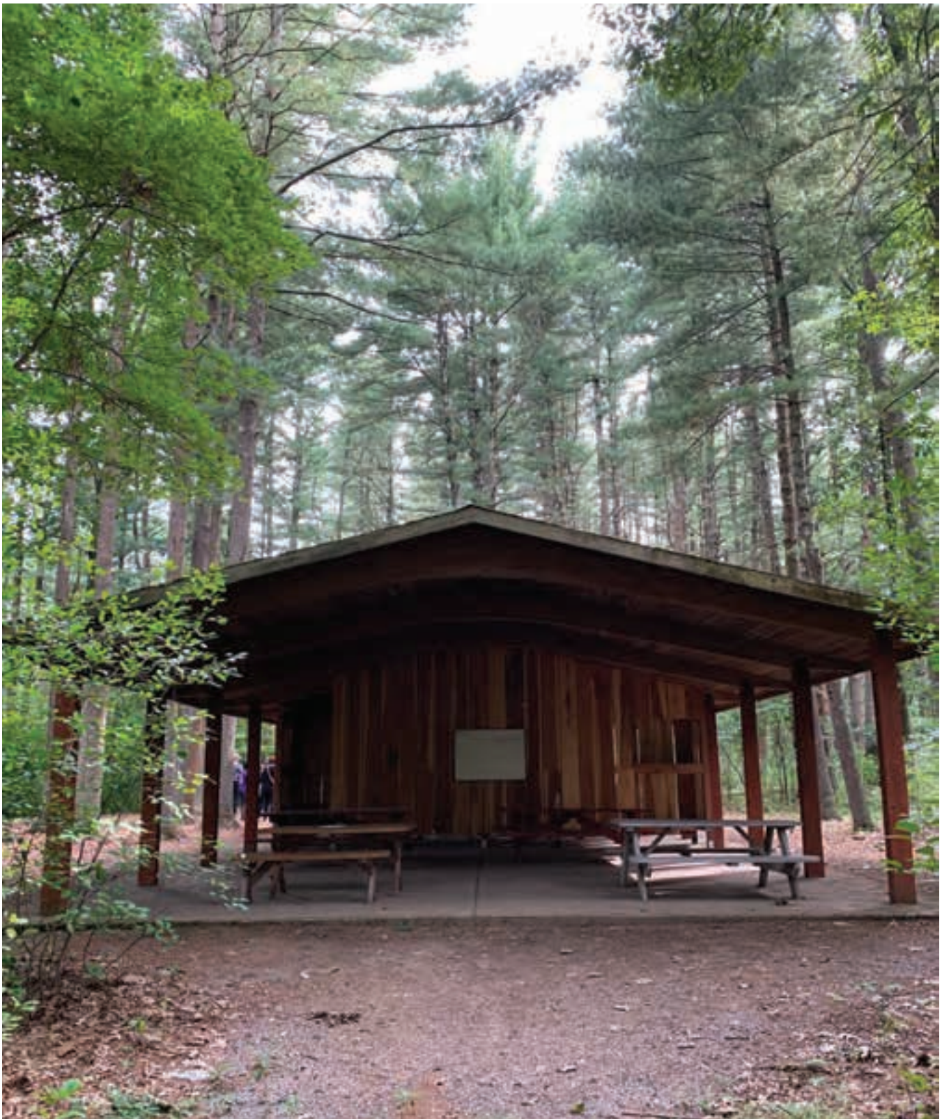
Figure 2-96. End elevation of a pavilion, showing a typical covered activity area with picnic tables. A lack of electric lighting creates dim conditions in cloudy/low light conditions.
