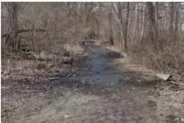
Figure 3-8. Trail is lower than the adjacent woodland causing runoff ponding on the trail and making it impassable.
