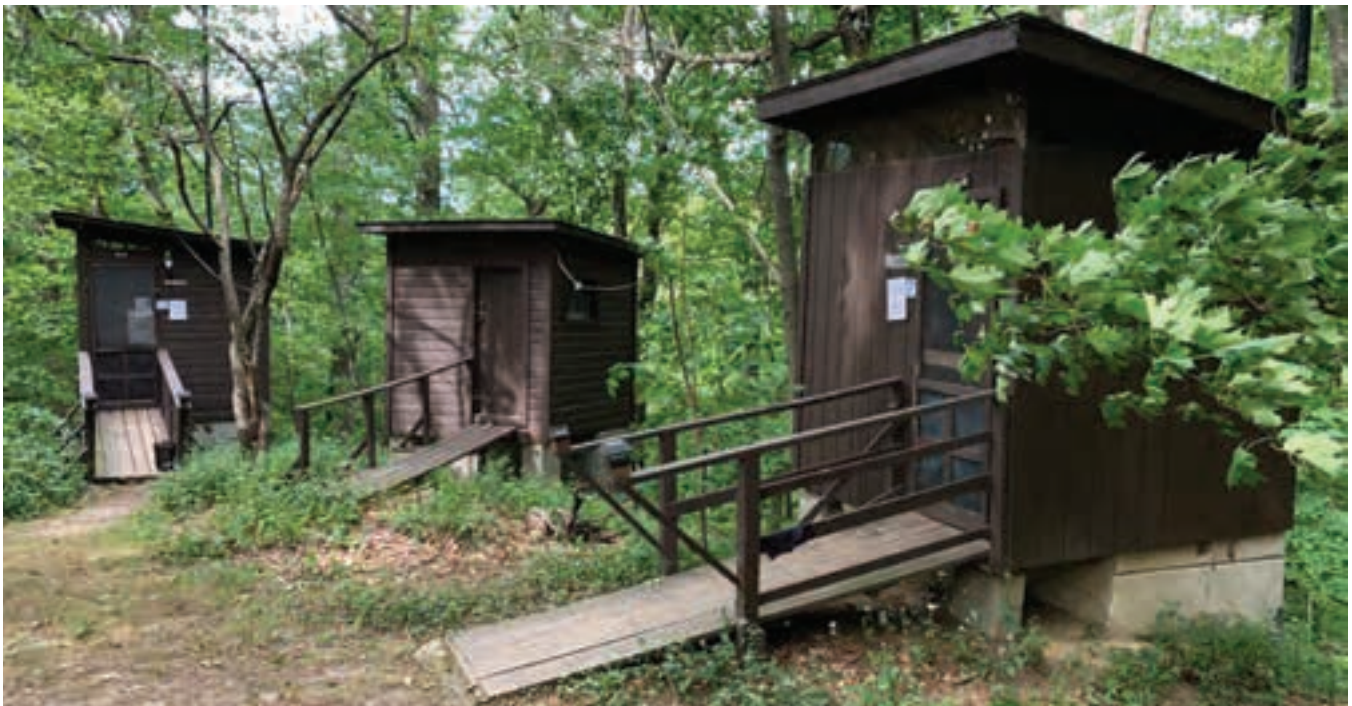
Figure 2-44. The Camp's restroom facilities, with men and women facilities at left and right and a storage shed is in the center.
