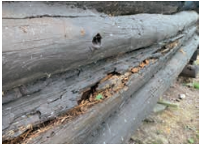
Figure 2-50. Evidence at Folsom of insect infestation within Chestnut logs
