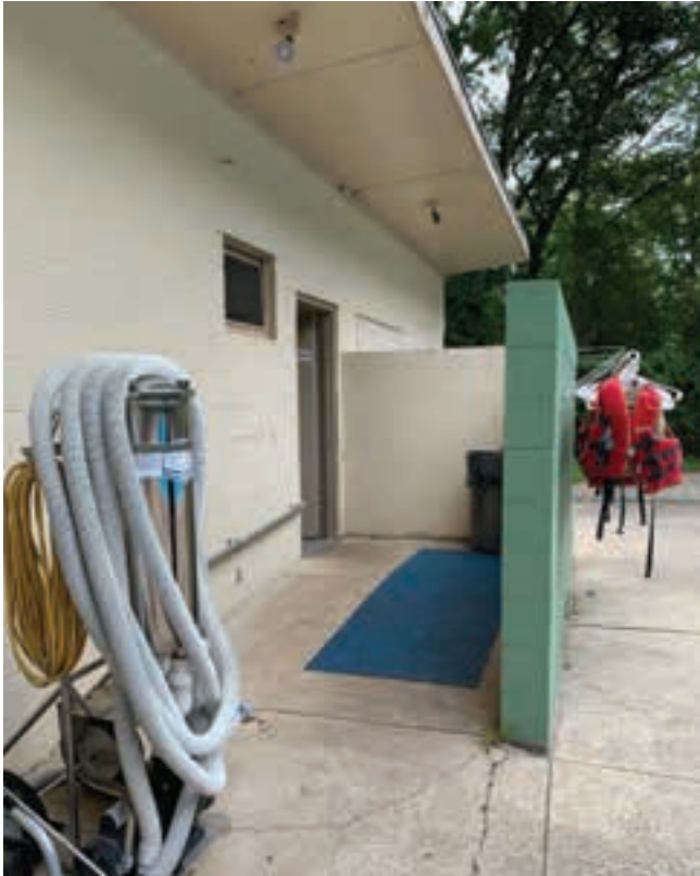
Figure 2-101. Restroom entry with a short, code-compliant ramp.
