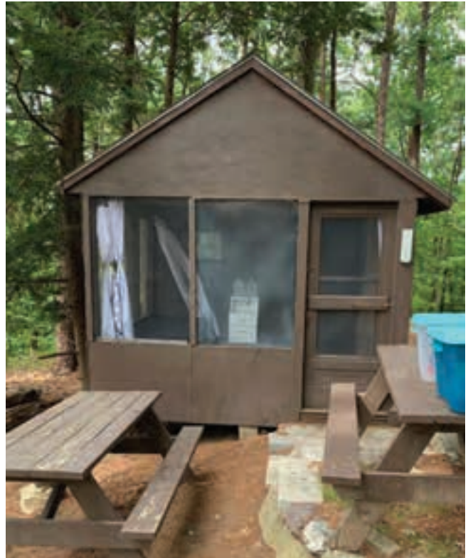
Figure 2-66. Smith cabin with stained plywood cladding
