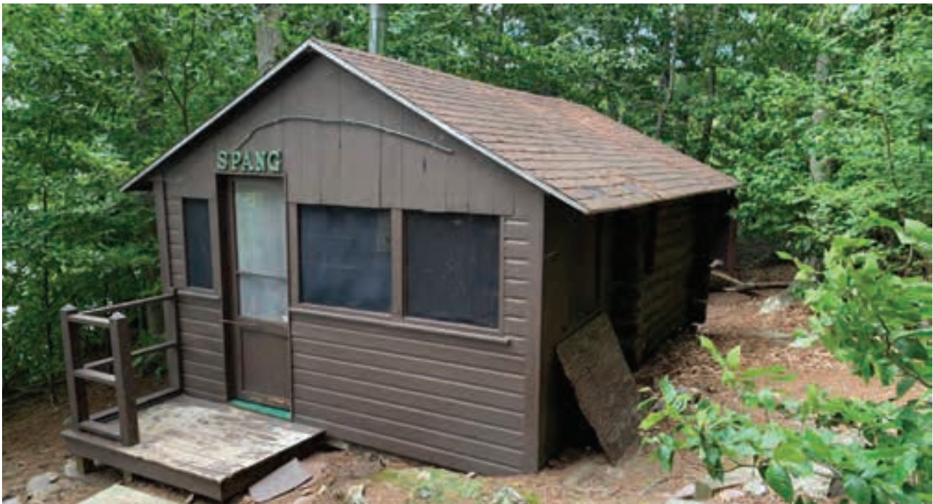
Figure 2-53. Spang cabin with the original log structure seen at rear.
