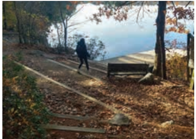
Figure 2-37. Stair and retaining wall at the swimming area
