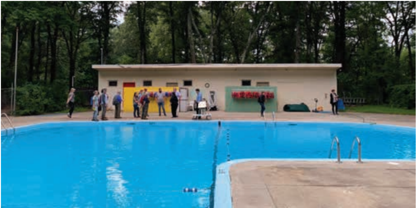
Figure 2-102. The YMCA Ponkapoag Outdoor Center's pool complex showing the in-ground pool, pool deck and bathhouse.
