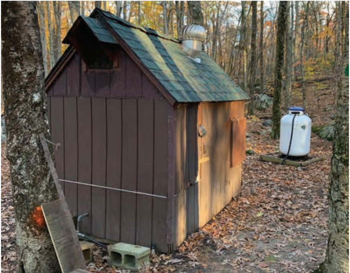
Figure 2-74. The Generator Shed with its remote propane tank
