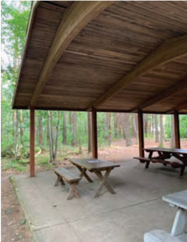
Figure 2-95. The pavilion's clear-span laminated timber structure
