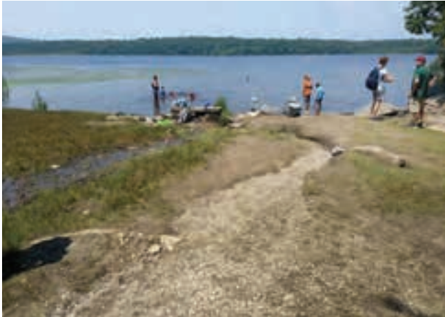
Figure 2-29. Rutting and erosion along the path all the way down to the water at Fisherman's Cove
