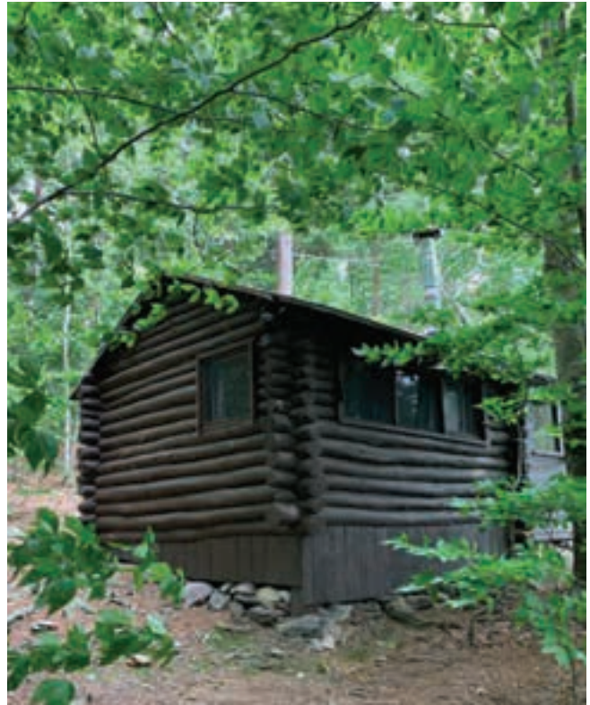
Figure 2-54. Spang's original log structure as seen behind its later front porch addition
