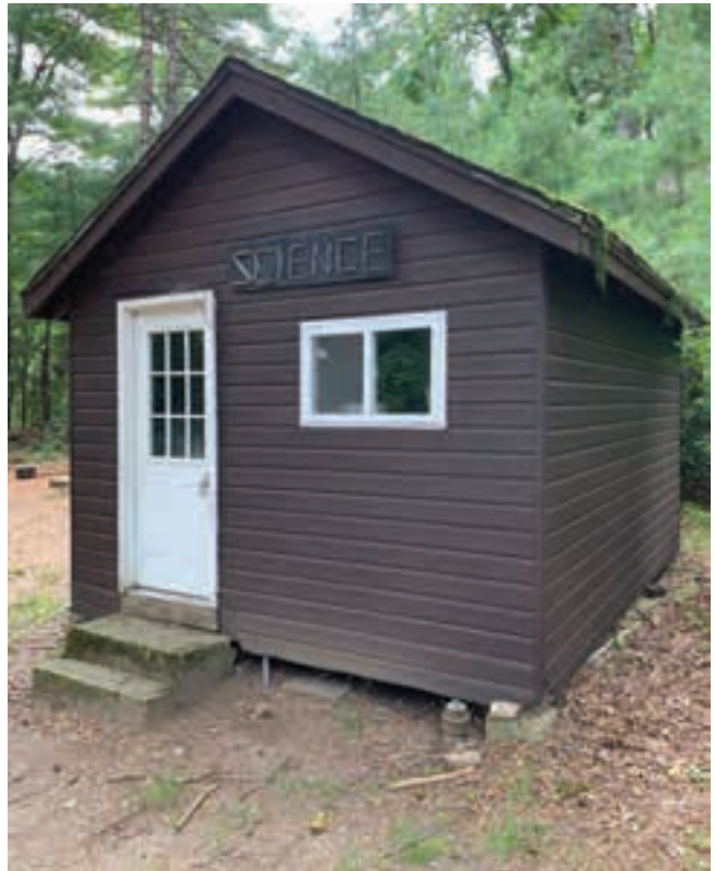
Figure 2-93. The Science Cabin's entry door.
