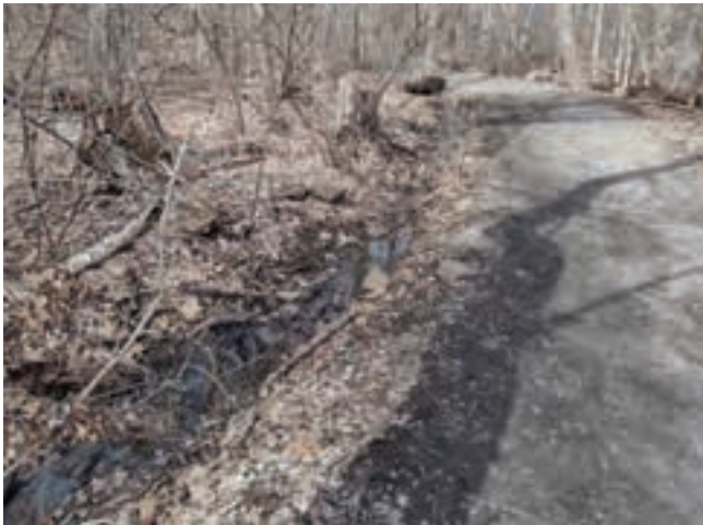
Figure 3-7. Vegetated swale along Green Dot Loop trail with a culvert at the low point to convey runoff to the other side of the trail.
