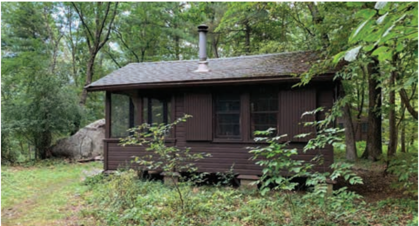
Figure 2-62. Duncan cabin's relatively flat site offers potential for an accessibility retrofit
