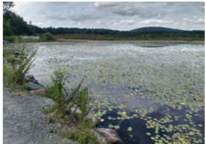
Figure 2-19. Open view at Dam
