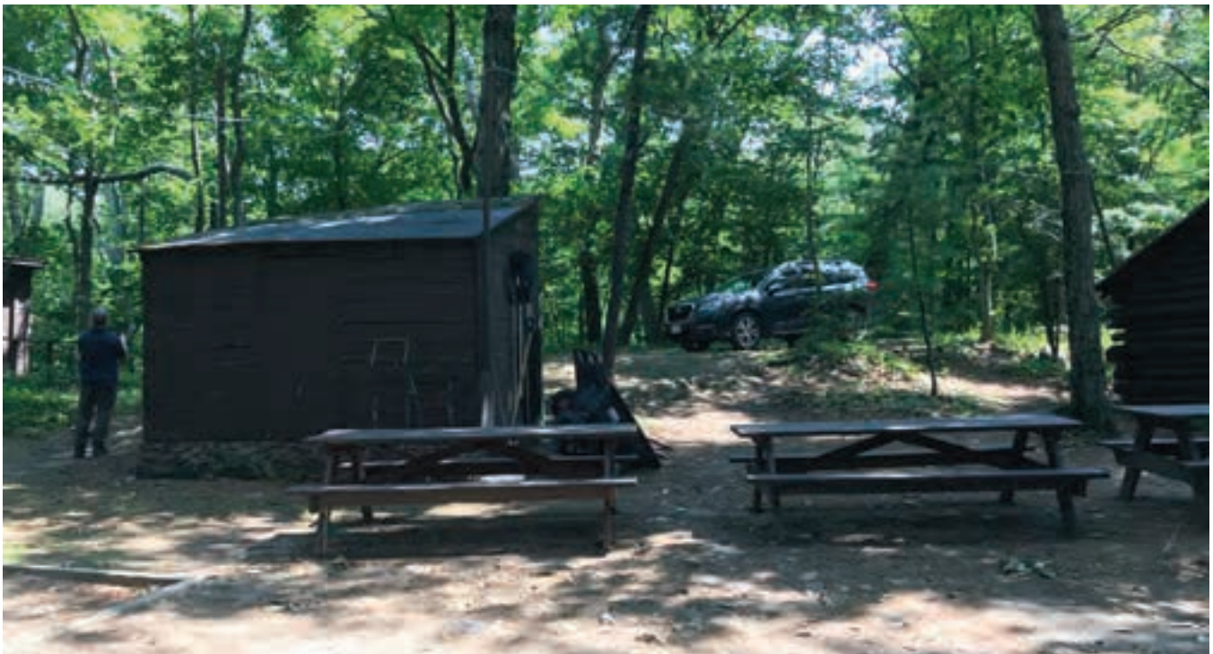
Figure 2-70. The storage building showing its stone foundation.
