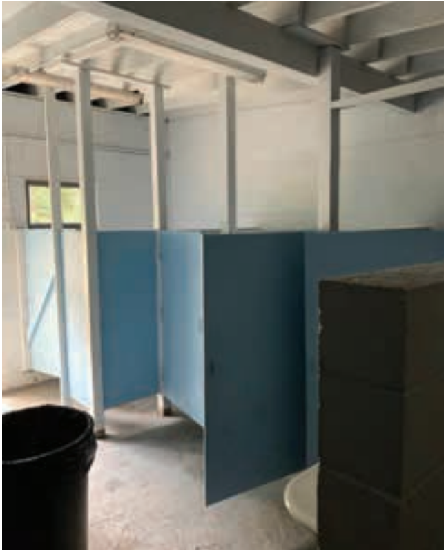
Figure 2-103. The restroom with wood toilet partitions.
