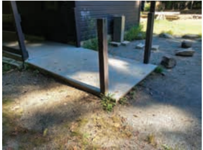
Figure 2-79. Non-accessible drinking fountain and restrooms
