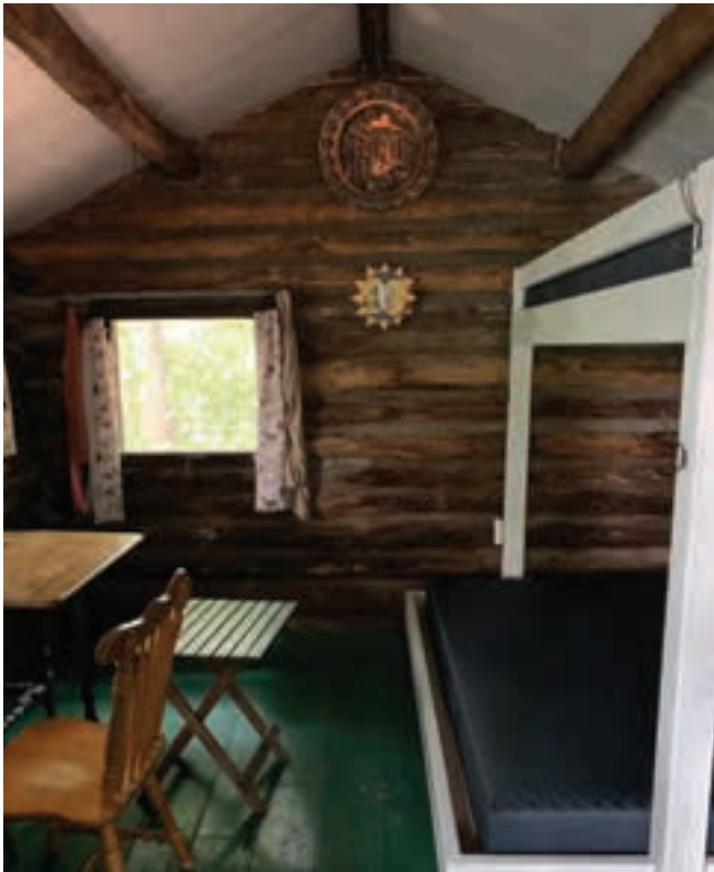
Figure 2-52. Spang's interior condition with exposed chestnut logs. Camp volunteers provide regular maintenance of the chinking between logs.
