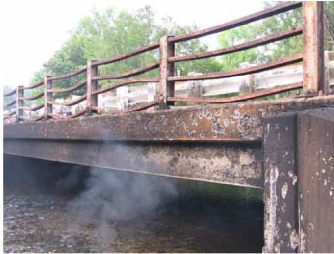
Figure 3.7: Fascia of Ridgefield, CT, bridge after the fire
