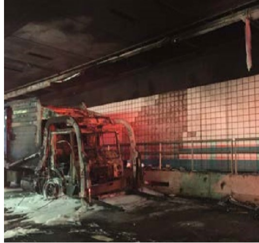
Wall tiles & lights (Temp. \geq 450^{\circ}\text{C} (842°F))
