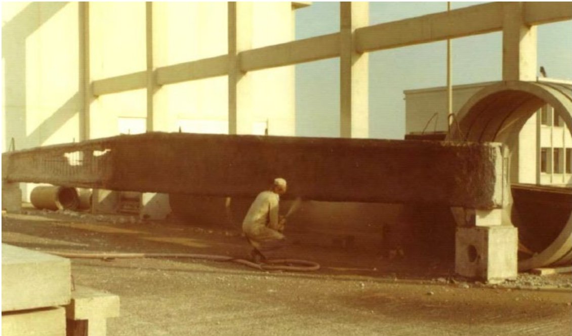
Figure 5.11: Application of shotcrete to damaged girder
