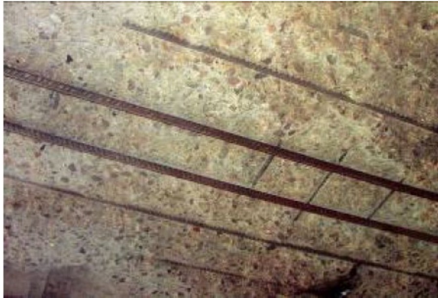
Figure 5.1: Buckled reinforcing bars in underside of slab
