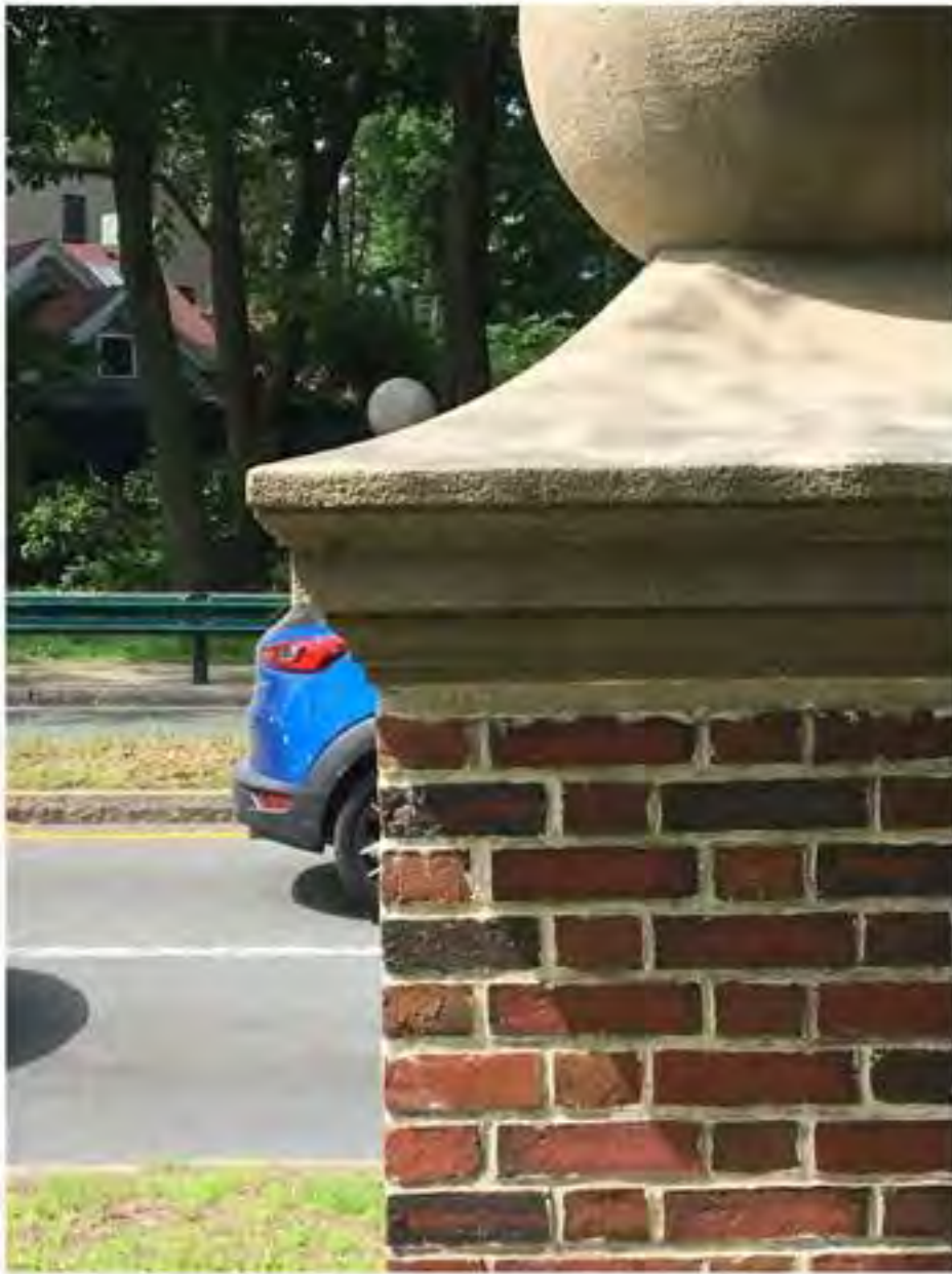
MIS-ALIGNED PIERS AT WEST SIDE
