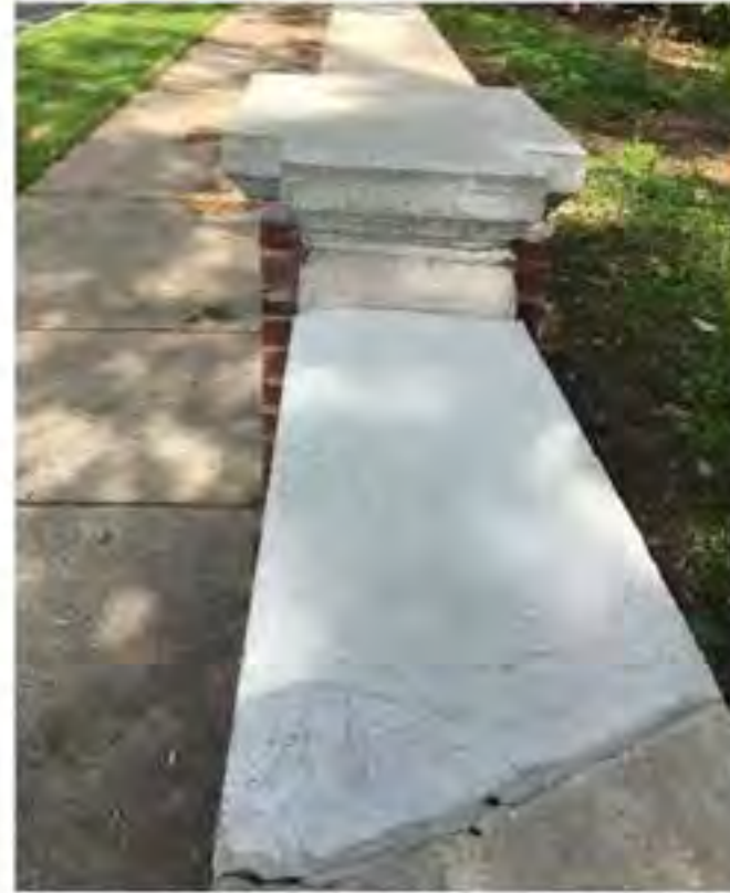
CAST-IN-PLACE CAPSTONE REPLACEMENTS
