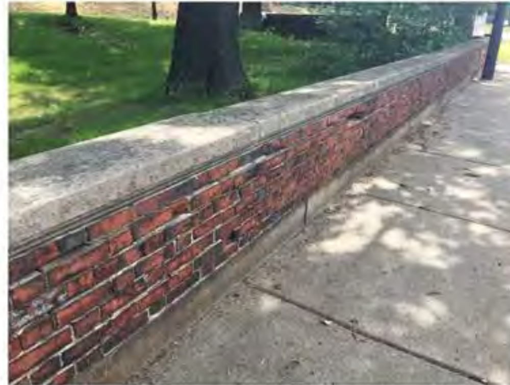
WALL CONDITIONS: MORTAR LOSS, MISSING BRICKS, LOSS OF FLASHING, CRACKING, ETC.
