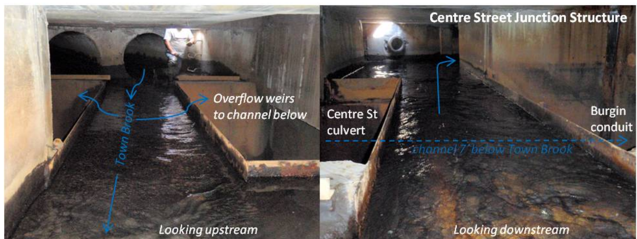
Figure 2.1-3 – Inside the Centre Street junction structure, looking upstream and downstream
