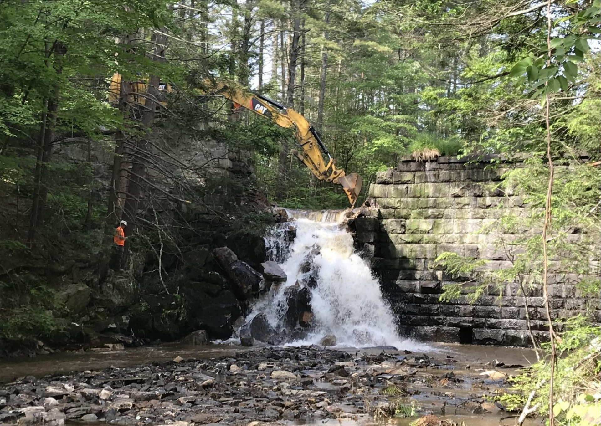
Recently completed Upper Roberts Dam Removal in Northampton
