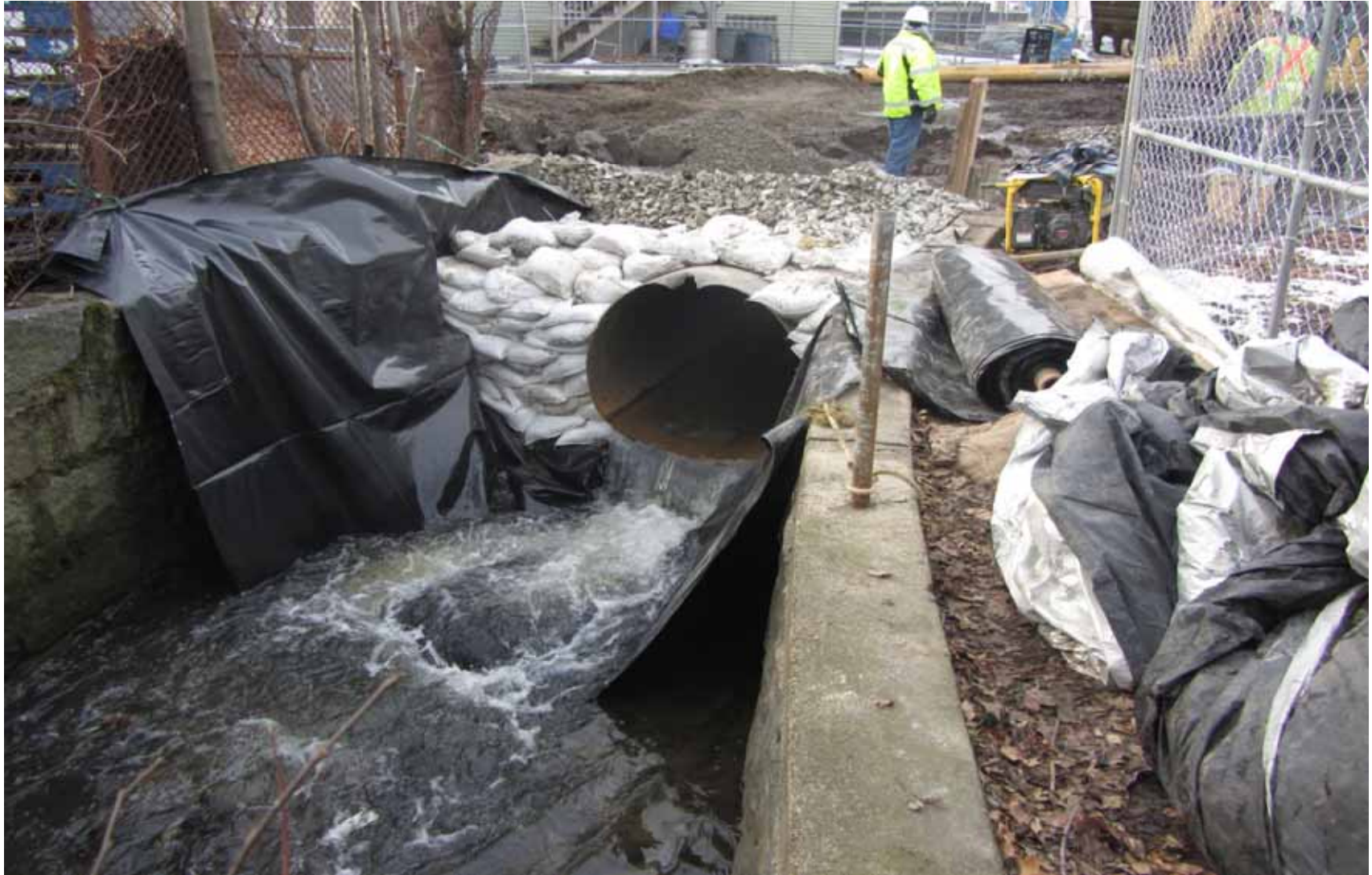
The existing Town Brook is temporarily placed in a culvert during construction. Note poly sheeting used for velocity dissipation at outlet.
