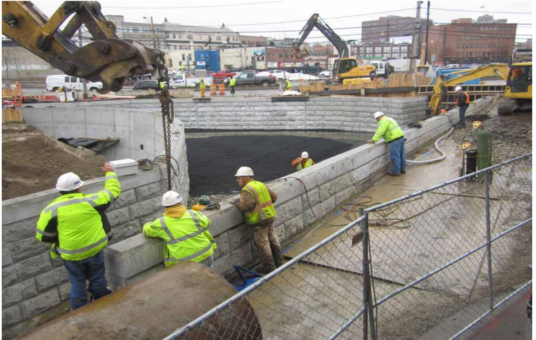
On March 6 th , the culvert carrying Town Brook was pulled and water flowed through the new alignment for the first time.
