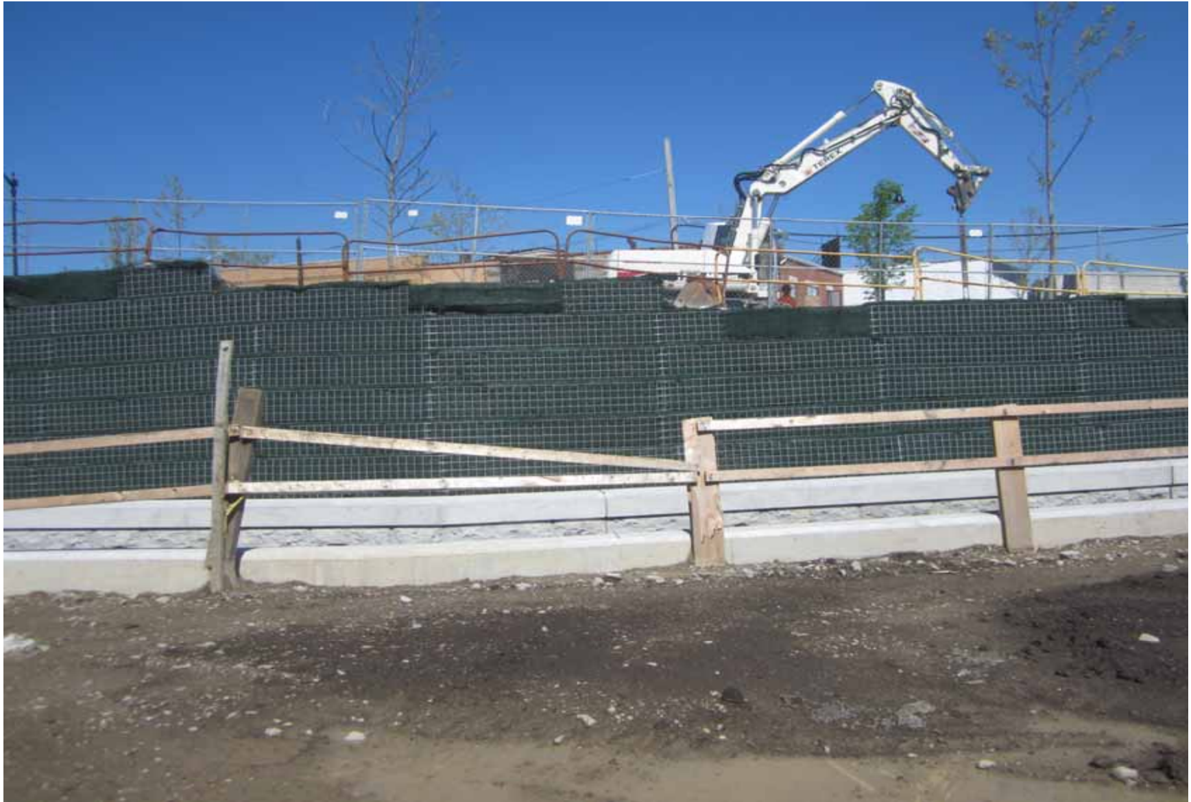
Construction of the vegetated retaining wall.
