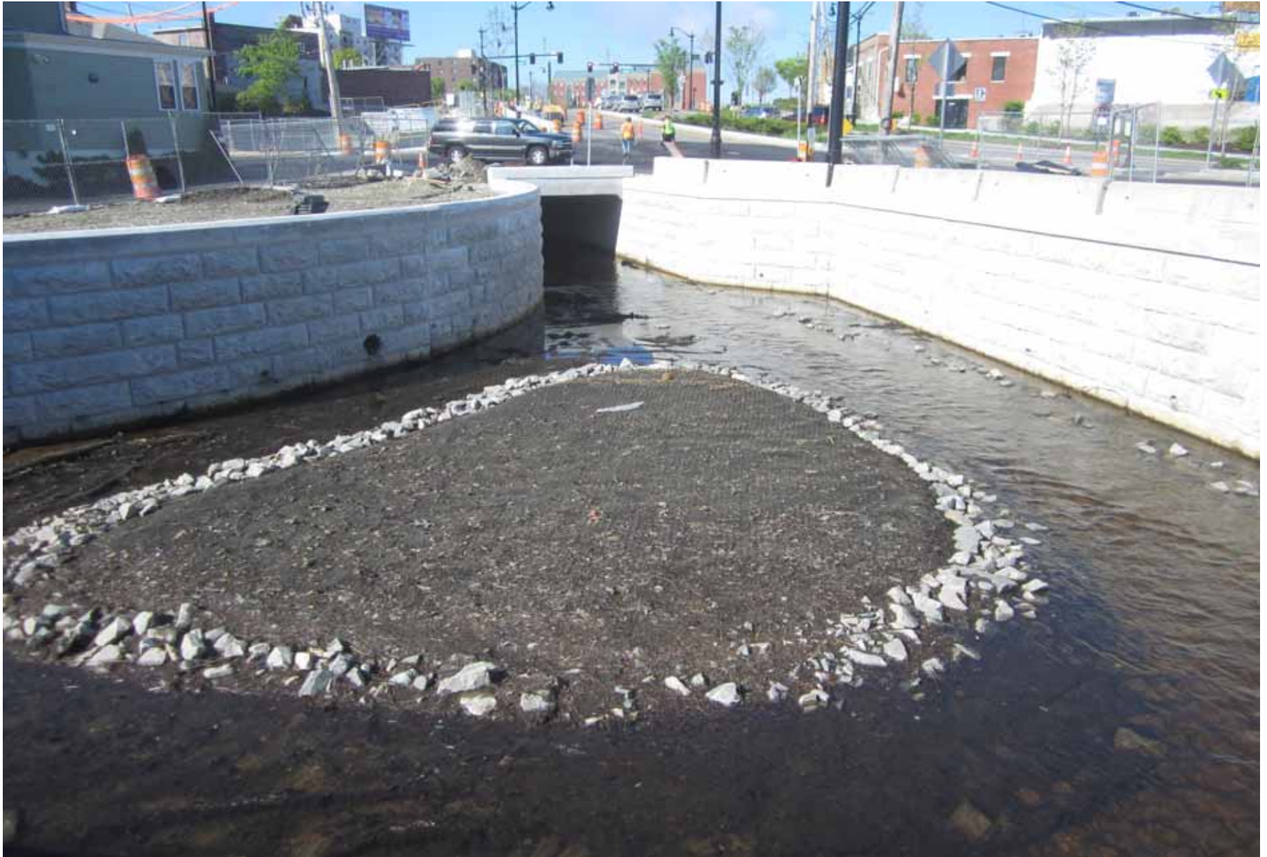
The toe of the BVW island was secured by stone as high flows were lifting the filter fabric.
