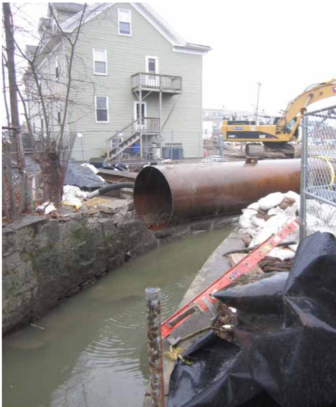
Culvert carrying Town Brook flows is removed.
