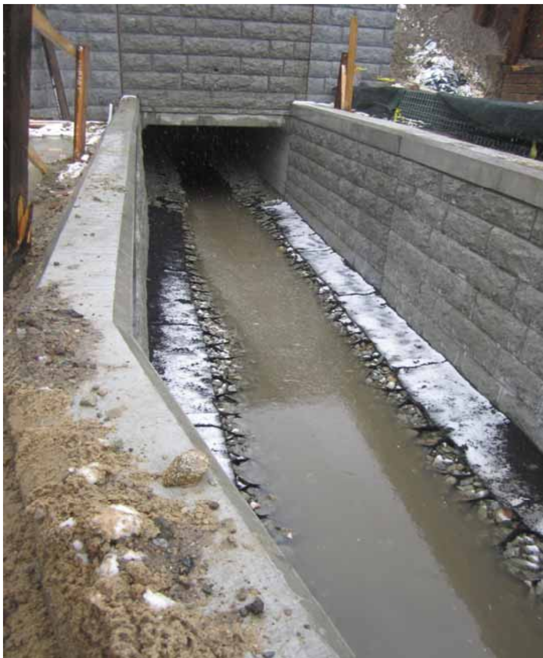
First flush as water flows through the new alignment for the 1 st time.
