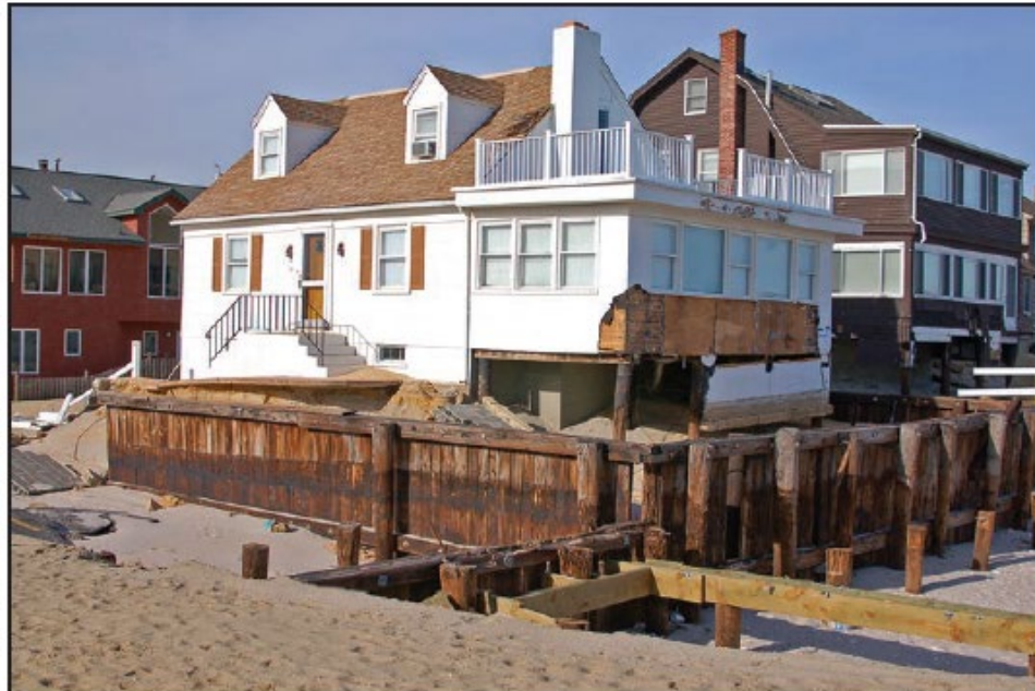
Figure 3-16: Timber bulkhead was overtopped, resulting in lost backfill and damage to the house situated approximately 15 feet landward of the bulkhead (Lavallette, NJ)
